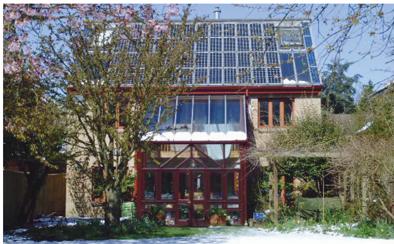
Susan Roaf's eco-house in Oxfordshire is one of the most high-profile low-energy homes in the UK
